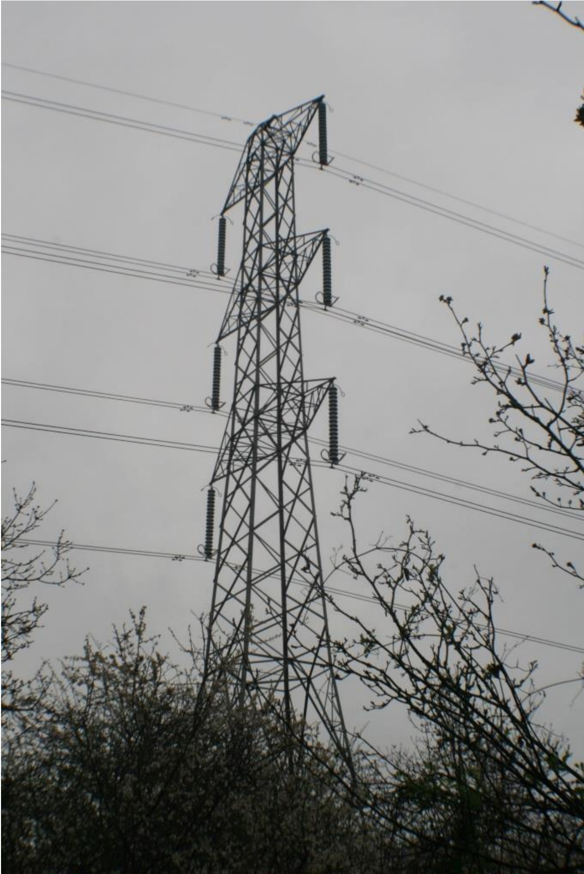
Electricity pylon within the land being purchased
